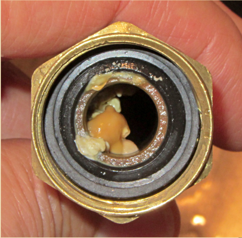
Microbial growth in a hot water pipe.
